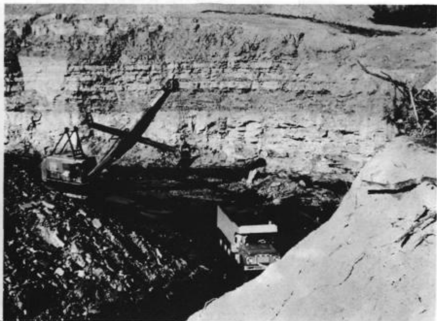
Figure 12 - Strip pit 1000 x 80 x 50 feet deep to serve as holding lagoon at Shannopin No. 1 air shaft treatment plant.
