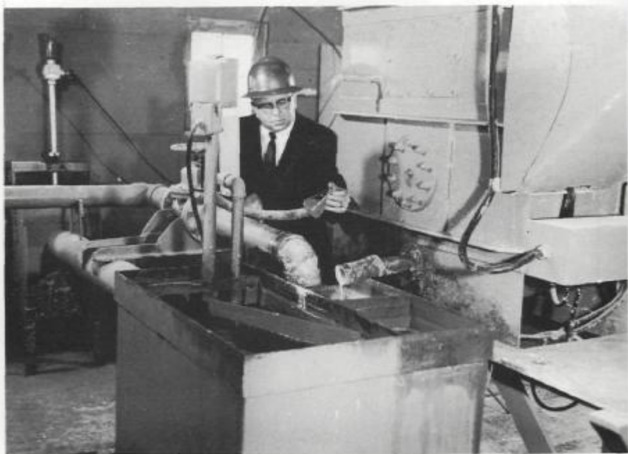
Figure 3 - Lime feeder and mixing tank at Thompson treatment unit. Note pH electrode in overflow line.
