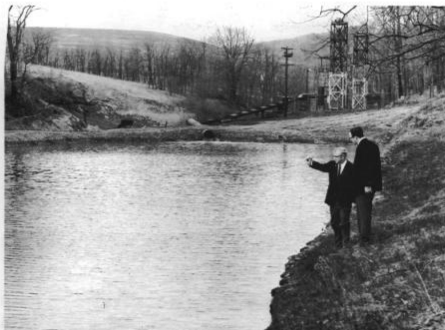
Figure 6 - First holding lagoon at Bercik Borehole, with discharge pipes and aerator in background.
