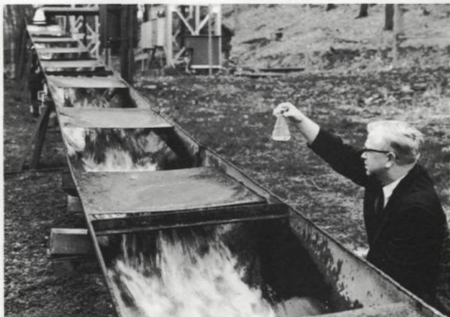
Figure 5 - Aeration trough at Bercik Borehole treatment plant, showing vigorous agitation in gravity flow.
