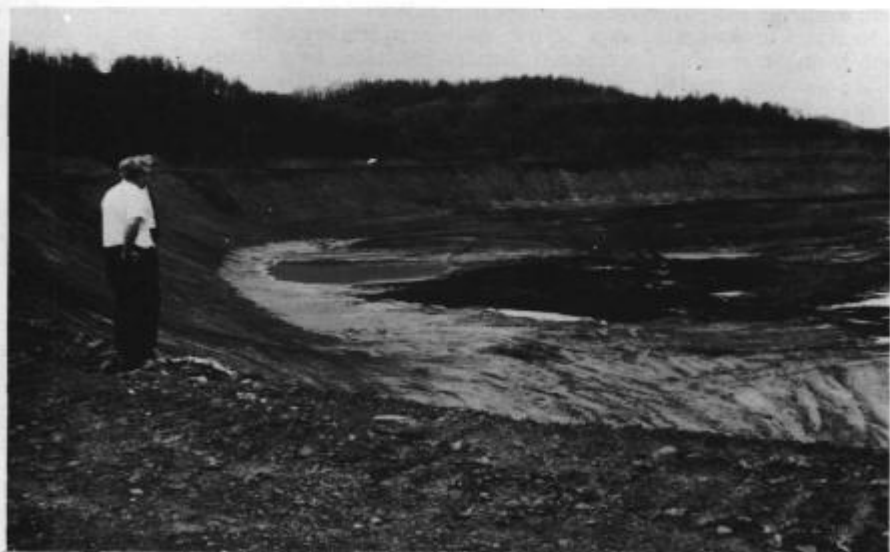
Figure 13 - Earthwork for diked lagoon to provide settling at Shannopin No. 1 air shaft treatment unit.
