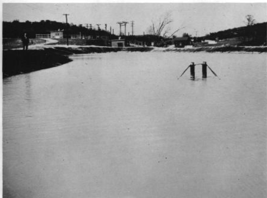
Figure 2 - 750,000 gal holding basin at Thompson Borehole treatment unit. Standpipes in center of basin control flow to neutralization unit.
