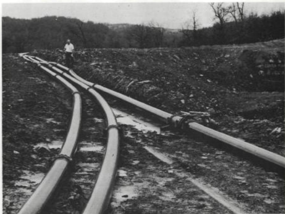
Figure 10 - Pipes from borehole to holding lagoon (left) and from holding lagoon to treatment unit at Shannopin No. 1 air shaft.
