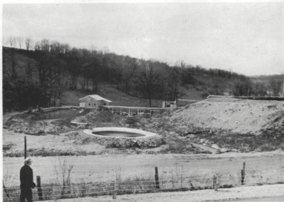
Figure 4 - Overall view of Thompson Borehole treatment unit. Holding lagoon at right, neutralization in building, settling lagoon with sludge pumps at left and fish pond in foreground.
